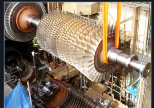
DRY ICE BLASTING IS IDEAL FOR MINOR OUTAGES PRE-INSPECTION CLEANING
