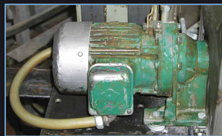
UNCONTAMINATED MOTOR AFTER UNDERGOING DRY ICE CLEANING
