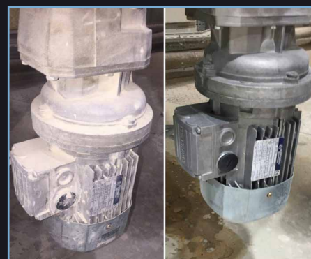
ELECTRIC MOTOR RESTORED AFTER DRY ICE CLEANING
