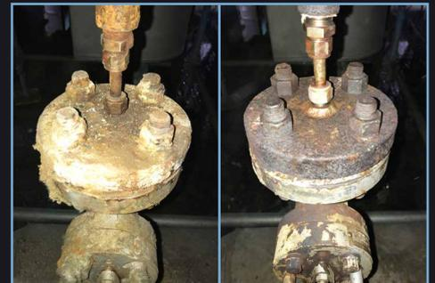
CONTAMINANT EFFECTIVELY REMOVED FROM A FLANGE AFTER DRY ICE BLASTING
